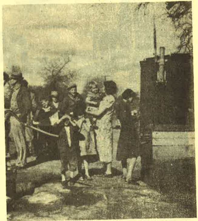
Workers in camp; note polluted water pool
