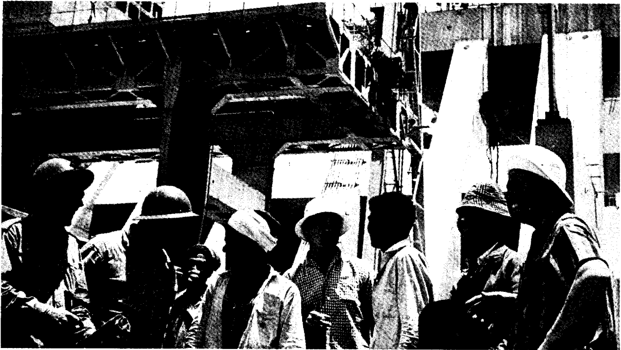
Soviet engineers, with Egyptian workers during construction of the Aswan Dam. The Soviets can afford to grin—as the text below shows, Soviet profits on the job were not just water over the dam.
